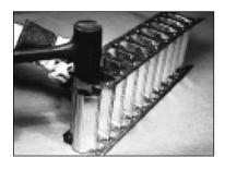
Assembly is ready to be inserted into the duct. Fasten to duct wall per the SMACNA recommendations.
